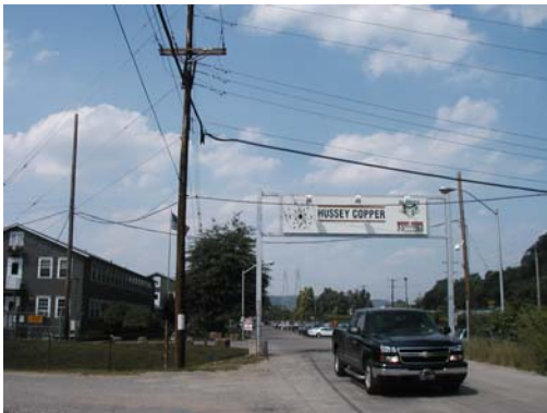
Entranceway to Hussey Copper constrained by utility poles to the left of the entrance and a sign that was too narrow to support the new turning radius required by delivery trucks.
