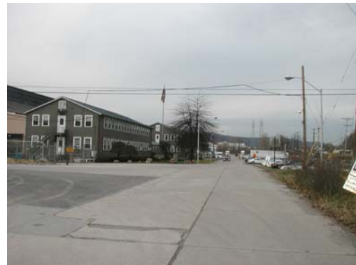
The new entrance configuration allows unimpeded access into the Hussey Copper site. The sign, utility pole, and drainage ditch were all removed to support the left hand turn into the plant.
